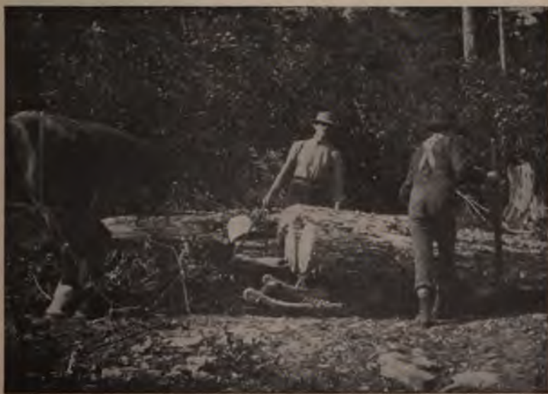
FIG. 33. — A Go-devil loaded with Hardwood Logs. Michigan.
